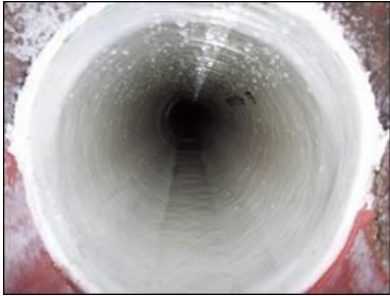
Cured in place pipe – lined pipe
