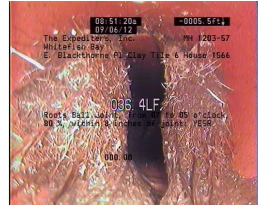
Root intrusion in a 6" lateral
