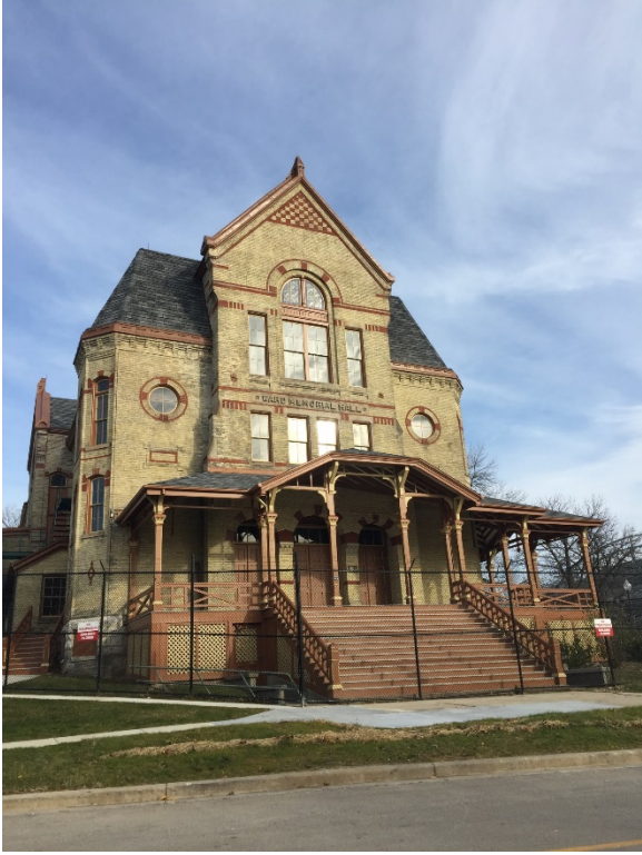
B41 Fully Restored Exterior
