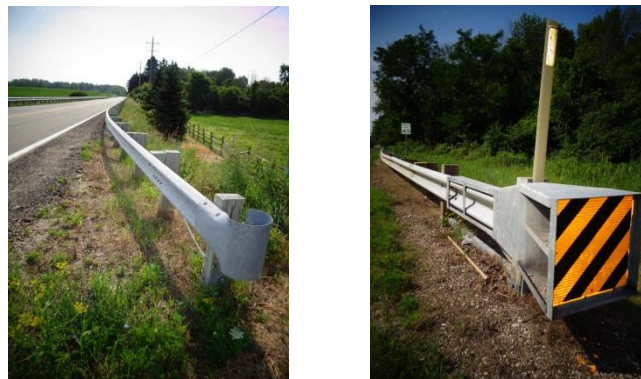
Figure 18: Guard rail end treatments
