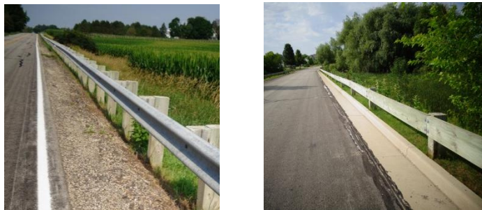
Figure 17: Metal and Wood Guard Rail
