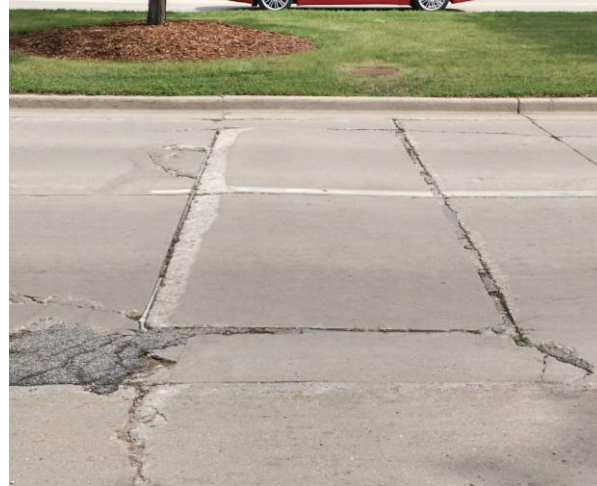
Figure 10: Loop Detector in Pavement
