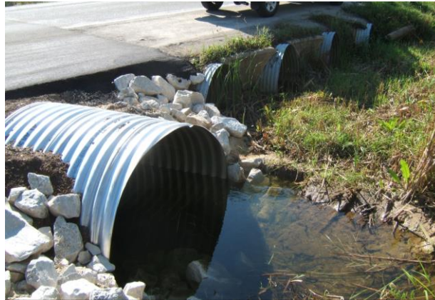
Figure 16: Multiple Cross Road Culverts
