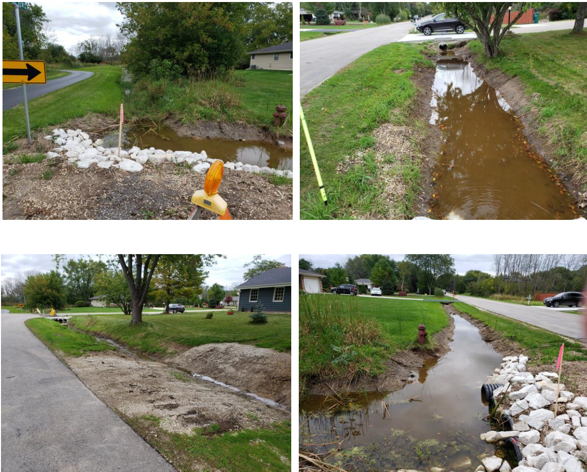
Figure 2 Photographs of North Prairie View Lane and West Revere Road in Mequon, Wisconsin Taken on September 21, 2021 by Anchor QEA
