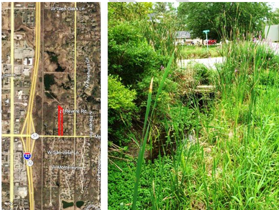
Figure 4. Map of study area showing location of proposed ditch modifications (left). Photograph of the existing ditch and culvert looking south towards Revere Road and Prairie View Lane intersection (right).
