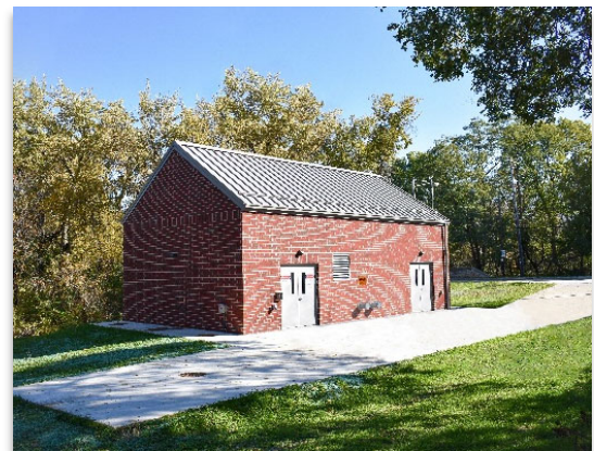
FIGURE 5-1 South Milwaukee North Chicago Lift Station
