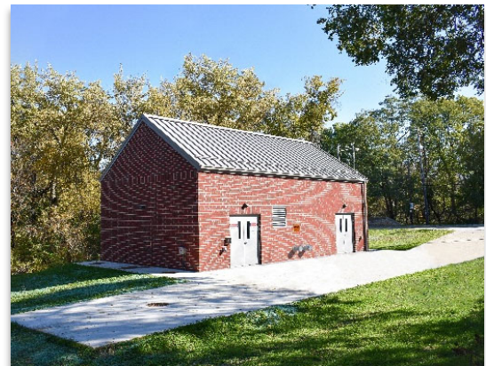
FIGURE 1-1 South Milwaukee North Chicago Lift Station
