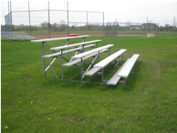
Bleachers should be on a concrete pad
