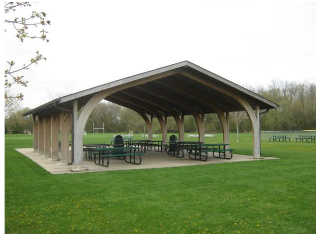
No ADA access to shelter
