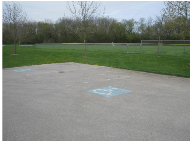
No ADA parking signage
