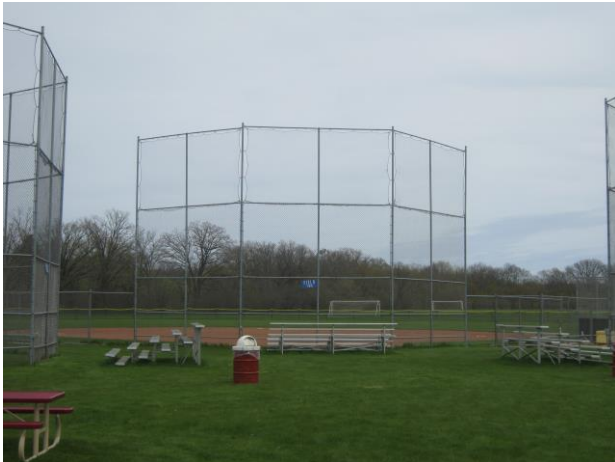
Bleachers not on concrete pads
