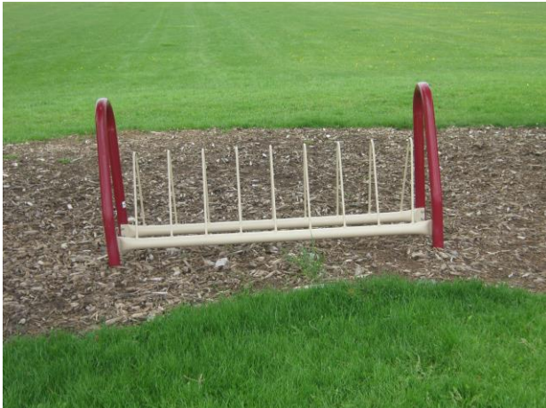
Bike rack is not on a hardscape surface
