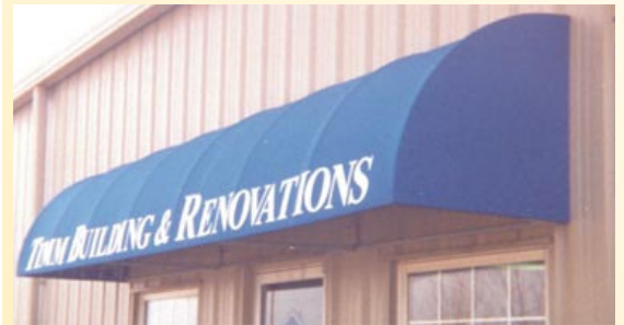
Undesirable Waterfall, or Bubble Type Awning
