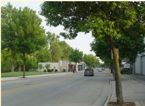
Existing South Main Street
