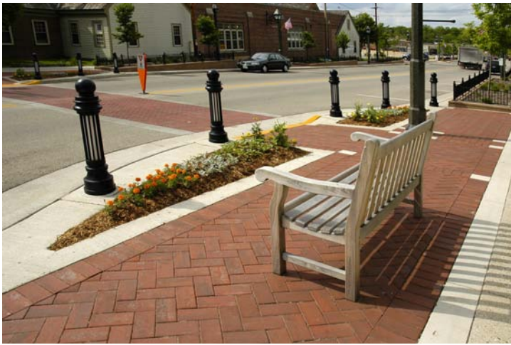
Enhanced Crosswalk and Brick Pavers
