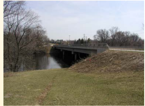
Milwaukee River Bridge
