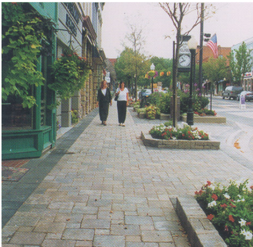
Paver Sidewalk and Planter Curb
